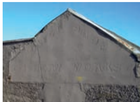
Figure 58 Gable end of a single-storey open-fronted curing shed. This was one of two concrete and corrugated-iron ranges built for the Tweed Fishery Works of Boston Brothers by Spittal builders A C Burns to designs dated March 1908. [DP071138]
